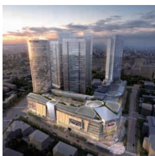
鄭州悅府 Zhengzhou MIXc Residence
