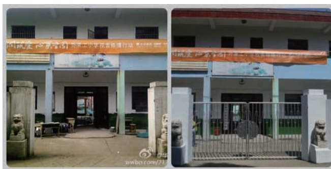
外來工小學校舍修繕 Migrant Workers Primary School Repairment
